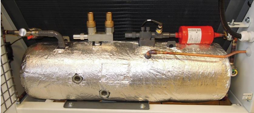
Figure 20: Liquid receiver with safety group
